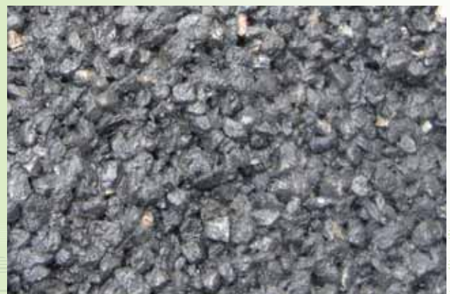
Bottom-layer after high pressure water cleaning and vacuum
