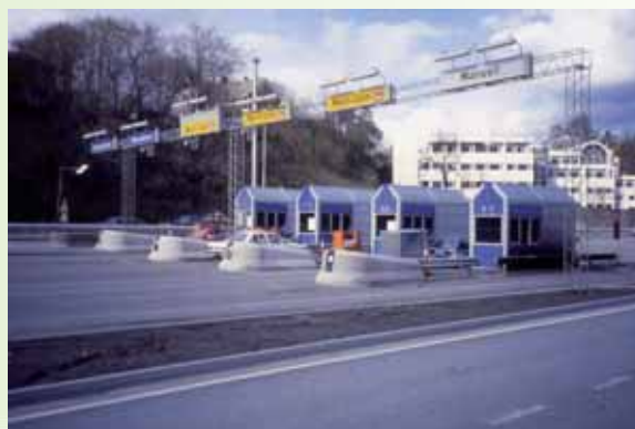
Congestion charge system in Oslo
